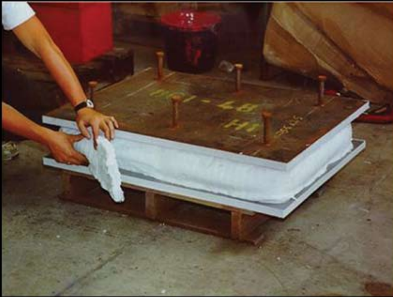
TICO ceramic fire blanket provides fire protection for bearing.
